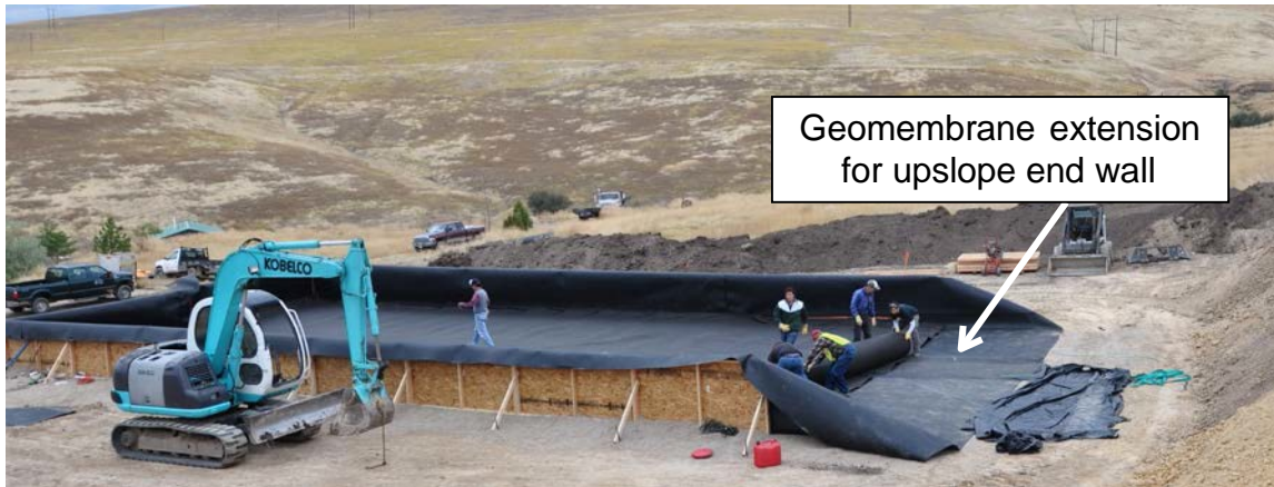
Figure 3. Geomembrane extending over downslope end wall (upper) and deployed out the upslope end of lysimeter for upper end wall (lower). (Photos courtesy of Dr. Craig H. Benson)
